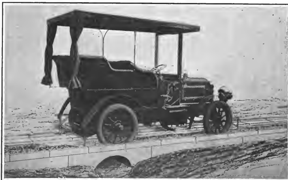
"MONOLITHIC RAILWAY" FOR AUTOMOBILES, DESIGNED BY J. V. GODMAN OF WARSAW, IND.
